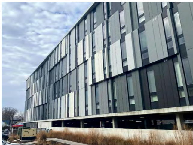
Exterior of 3435 Main - KC's First Modular Apartment
