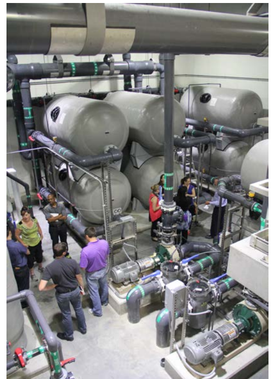
Exploring the Penguin exhibit pump room.
