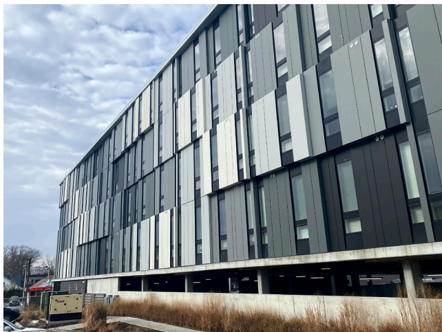
Exterior of 3435 Main - KC's First Modular Apartment
